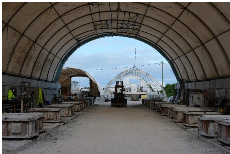
Above: The Precast Concrete Aust manufacturing facility at Pinkenba, Queensland
