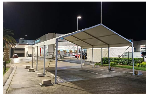
Concrete blocks used to anchor marquees
