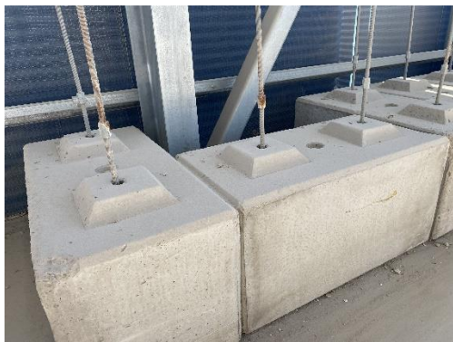
Building Protection composed of interlocking concrete blocks
