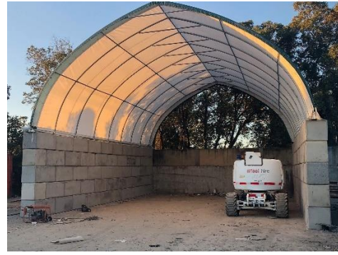
Igloo/Dome Structure Support constructed from interlocking concrete blocks
